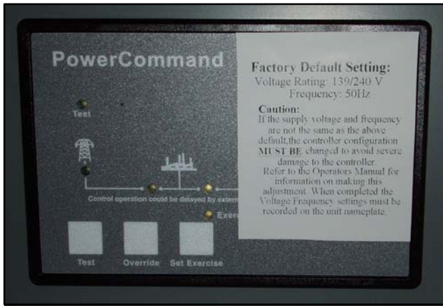
FIGURE 7-17. FACTORY DEFAULT SETTING LABEL ON CONTROL
