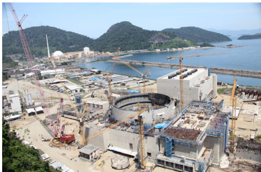
Figura 1.8 – Usina nuclear de Angra 3.
